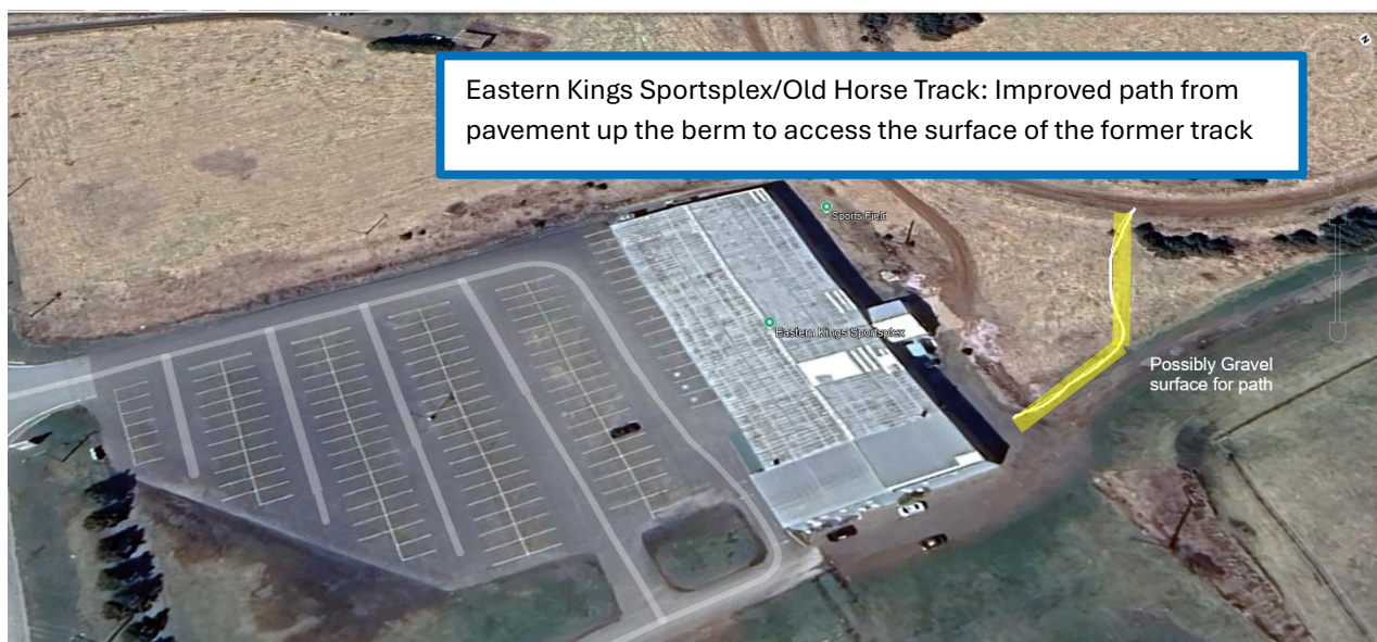
Photo 5 – Potential connection from pavement to the former track surface.
